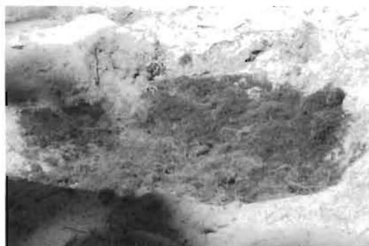
Fig.10. Coir pith applied in the pit
