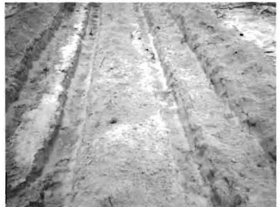
Fig.1. Opening of trenches
